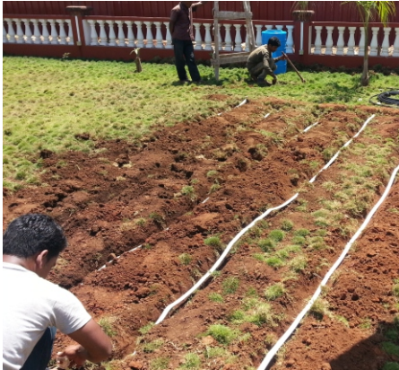
Installation of Moistube at a gap of 2 feet each, in a 4 inch deep trench in an area of 180 sq. ft
