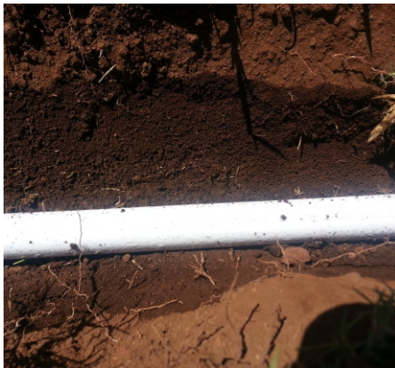
Water being absorbed by the soils capillary action
